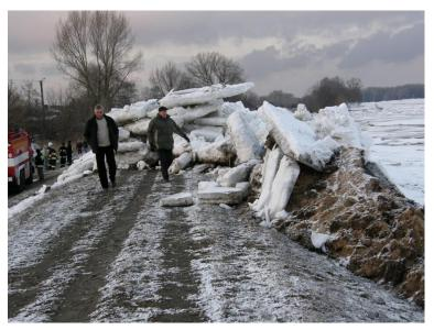
Figure 6.16. Ice-jam on the Vistula near Płock (04.03.2010) – damaged embankment at km 597
